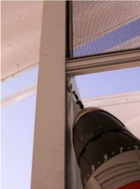
Choose where you will drill the holes before you do it. There are two considerations here. First you must make sure the spoke will not interfere with the retaining latch on the main door.
