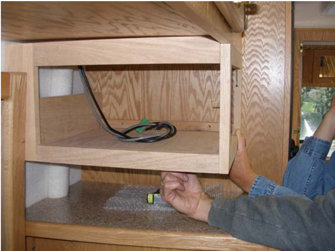
Fitting the new cabinet and shelf.
